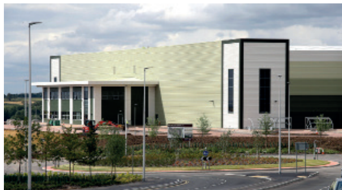
Firemac Project: Amazon Warehouse, Rugby
